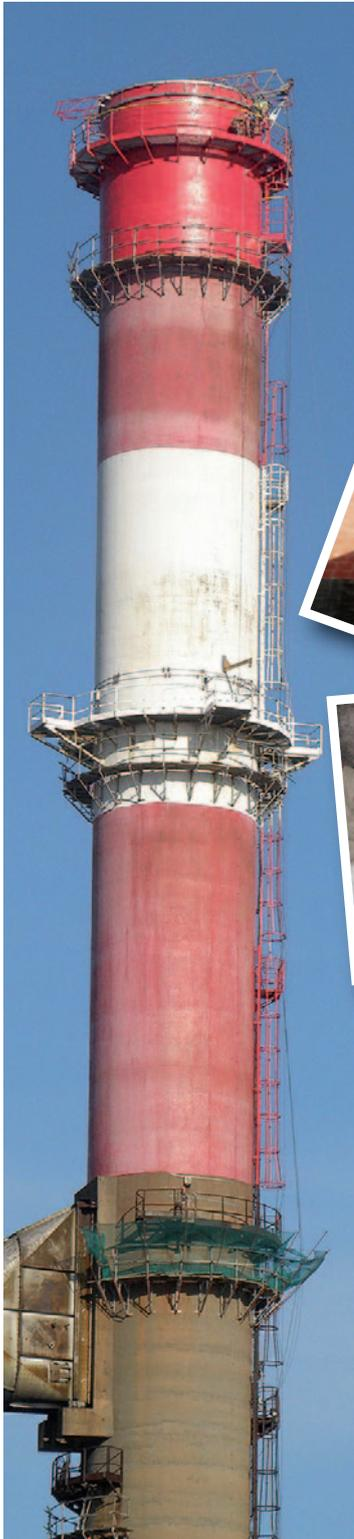
During a plant shutdown, FERBECK INDUSTRIAL CHIMNEYS has been in charge of the full refurbishment of a concrete stack including: brick liner replacement, installation of new accessories such as ladders and platforms in order to comply with new European standards, external painting, new lightning protection system and new aircraft warning system.
