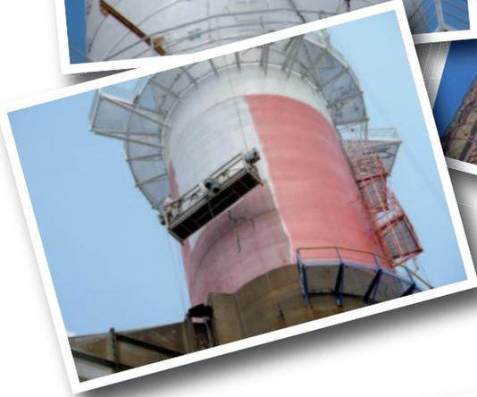
*Carrying out of the works in optimum security conditions: use of temporary platform with lifeline and external man baskets, discharge of the demolition wastes by external chutes...*
