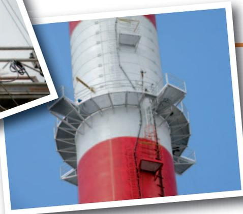
*The ladders and the platforms have been replaced by new ones, in order to comply with the norms.*
