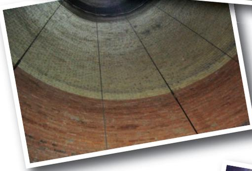
Sometimes, it has been necessary to replace additional full brick segments not included in the original scope of work. Then, FERBECK INDUSTRIAL CHIMNEYS showed its adaptation capacity and its faculty to react quickly by supplying immediately the complementary materials and to finish on time in spite of this unforeseen works.
