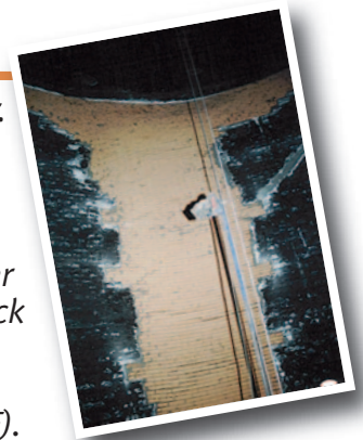
Insertion of a stainless steel inner liner in a steel stack.
