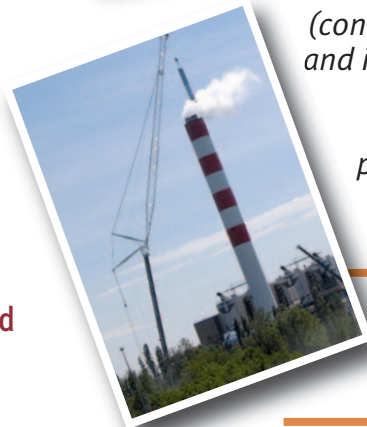
Insertion of a stainless steel inner liner in a steel stack.
