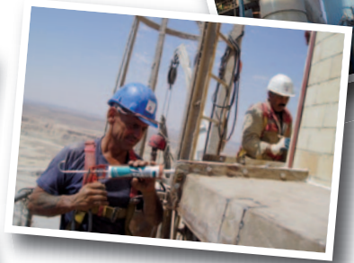
Complete refurbishing (concrete shell and inner brick liner) of a 140 m high stack for a steel producer in France.
