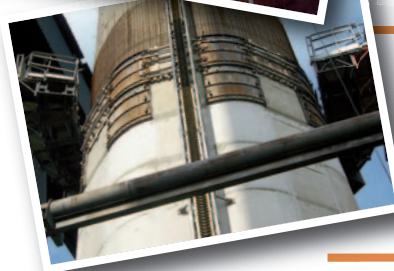
Complete refurbishing (concrete shell and inner brick liner) of a 140 m high stack for a steel producer in France.
