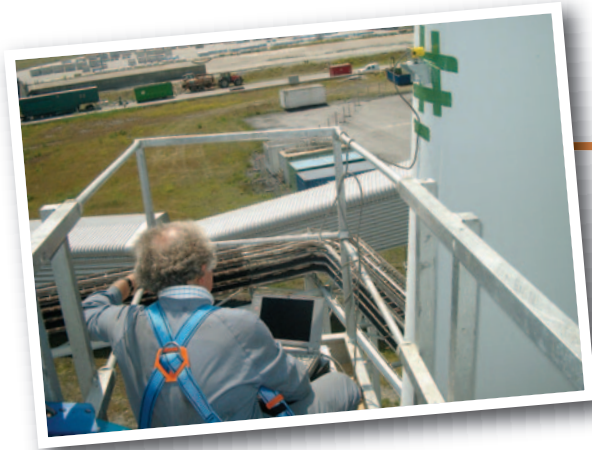
Lifting a special box with 4 videos for an on line hot video inspection.
