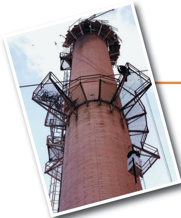
In situ vibration measurements prior installing an anti vibration damper.
