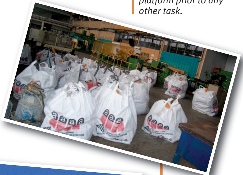
Polluted bricks have been packaged in big-bags for specialized treatment plant.
