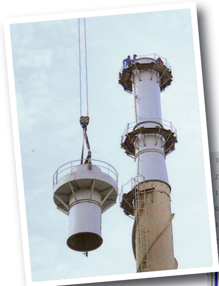
Installation of a damper on an existing chimney.
