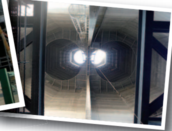
Construction of a 100m high concrete stack with two internal steel liners for a new power plant in Italy.
